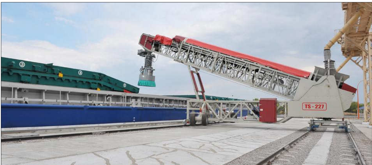
Figure Two - Mobile Ship-loader on rails moving parallel down quayside to next discharge point
