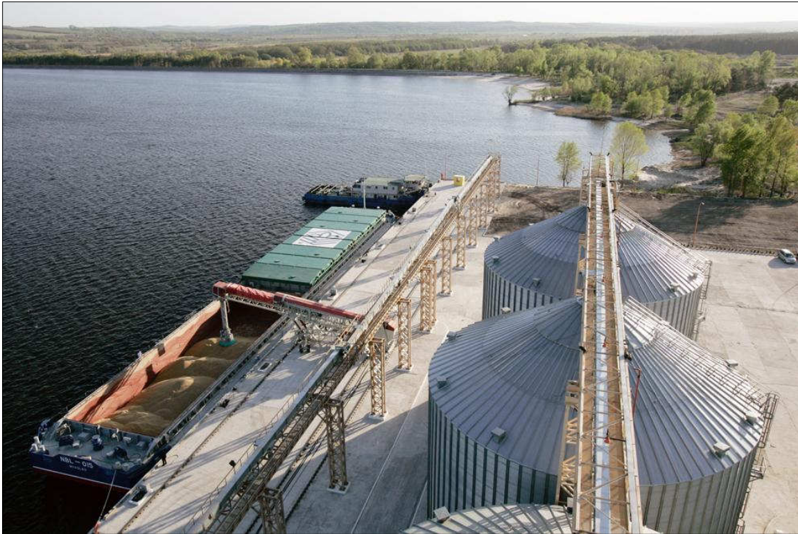
Figure Three - Mobile Ship-loader loading barges directly from grain silos
