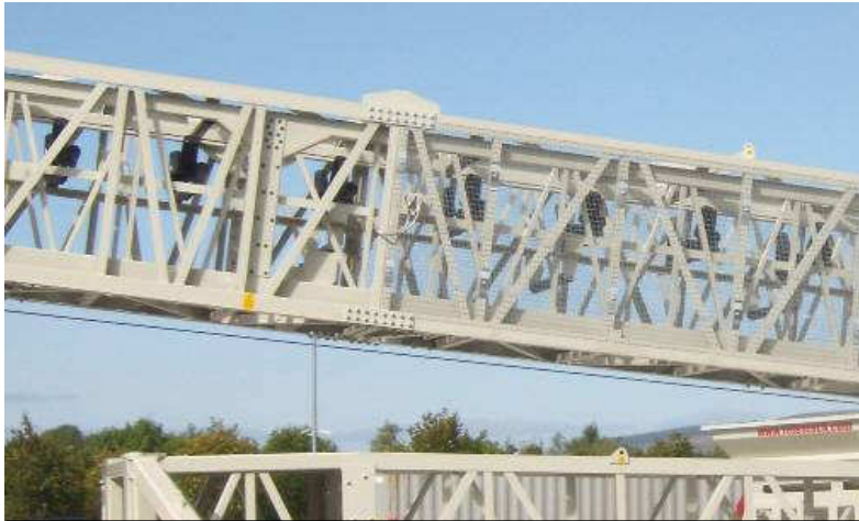
Bolted Sections (No welding)
